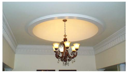
Imperial Measurement Outside Diameter 80" Flange 5" Inside Diameter 70" Inside Height 15" Material Thickness 1-1/2"
